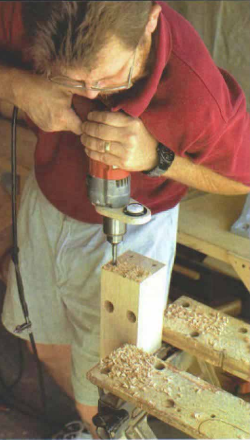
Bubble level keeps the drill straight. After drilling access holes in the newel, the author clamps the post plumb and drills four bolt holes that must be true. The bubble level's plywood base fits tightly onto the drill's motor housing.
